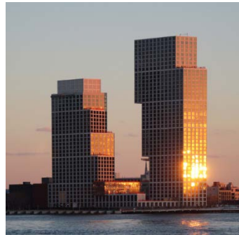
Eagle + West (New York, USA) 16 elevators
