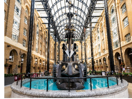
Hay's Galleria (London, U.K.) 9 elevators
