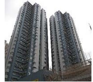
Walton Estate (Hong Kong) 12 elevators
