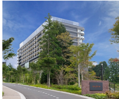
Fuji Speedway Hotel (Shizuoka, Japan) 10 elevators and 2 escalators
